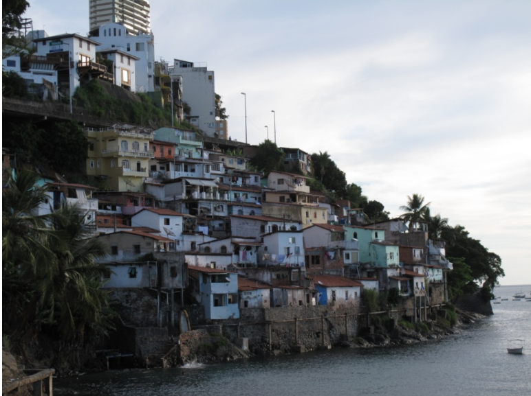
Photo 6. A condominal sewer scheme in a hillside favela on the coast in Salvador de Bahia
