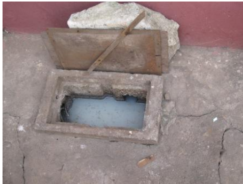
Photo 5: Grease trap in Kumasi, Ghana
