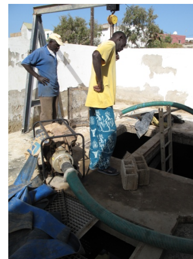
Photo 8: Emptying a lift station using a booster pump (Dakar)
