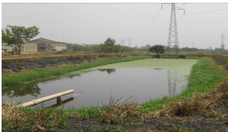
Plate 8: Additional anaerobic pond constructed to cater for institutional connections (Kumasi Polytechnic). Available land around ponds should be preserved against encroachment and for future expansions.
