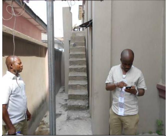
Plate 2: Well-constructed steps led to pan-latrine chambers on upper floors of tenement houses in Asafo.
